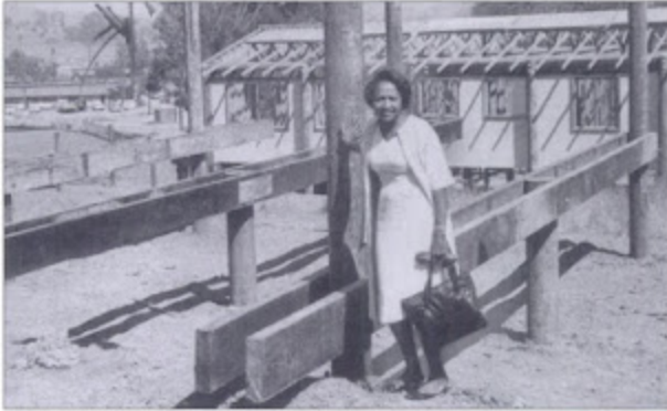
Although the developer initially promised fancier homes to Marin City inhabitants, residents dubbed the final offering "pole houses" because they were built with telephone poles. The county newspaper took this photograph of a local resident, Mrs. Moses Brand, outside a home under construction in 1962. (Photo courtesy of the San Francisco Public Library.)
